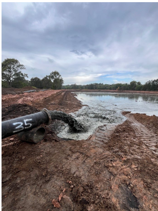
Photo 1: Pipeline testing and commissioning at Ningi DMMF
